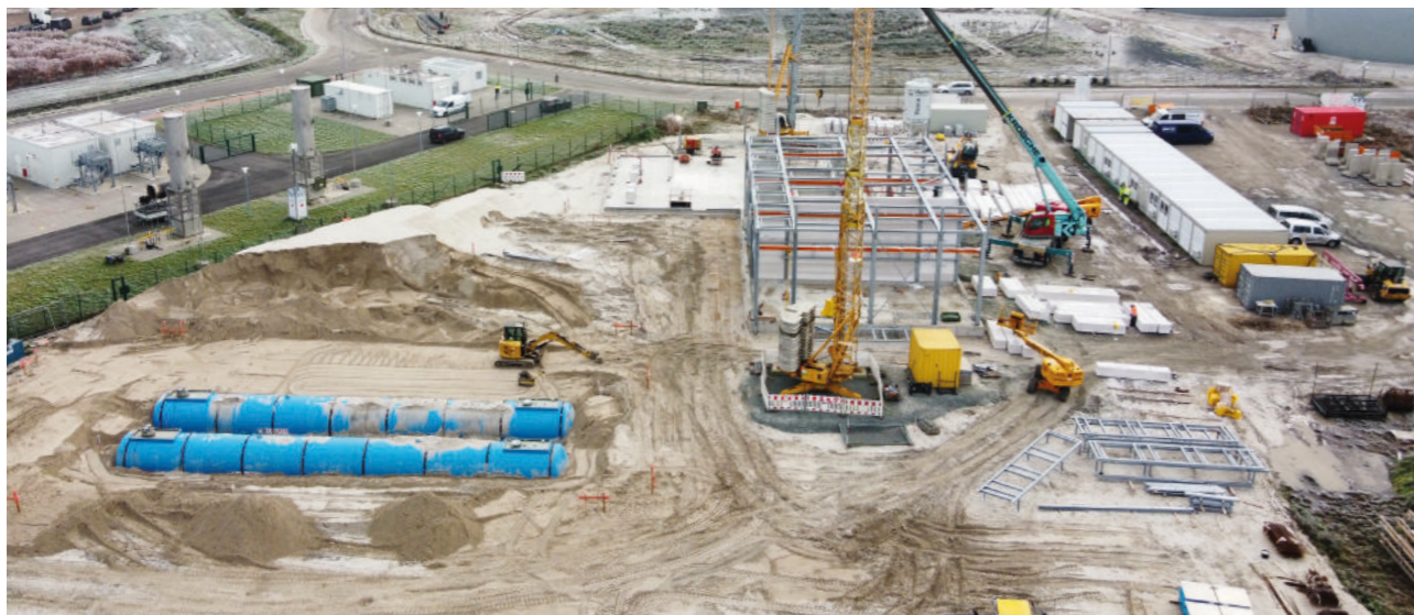
Approximately 50 systems built or delivered in the last 15 years.
