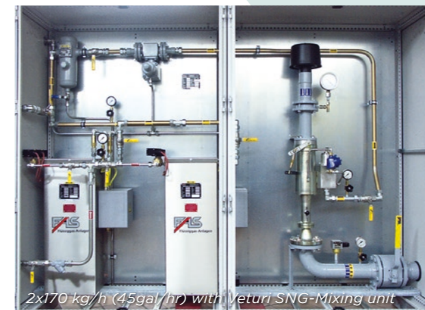
Waterbath vaporizer unit with redundant pressure regulation and electronic liquid level alarms.
